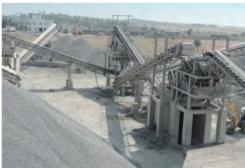
RAP Crushing & Screening Plant in Ethiopia
