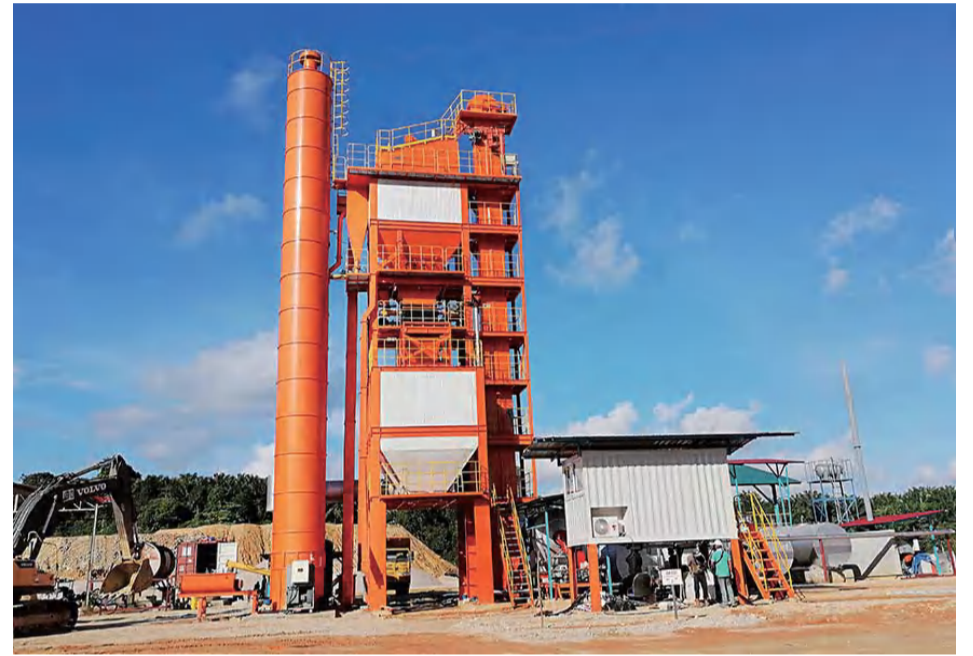
120TPH Asphalt Plant in Malaysia Won Client' s Praise
