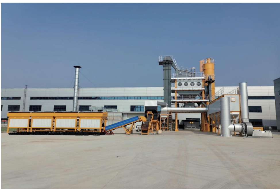
LB Asphalt Batch Mixing Plant in Nigeria
